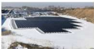
A 500 kW floating array located in Bayou County, where temperature can be less than minus 20 degrees Celsius.
