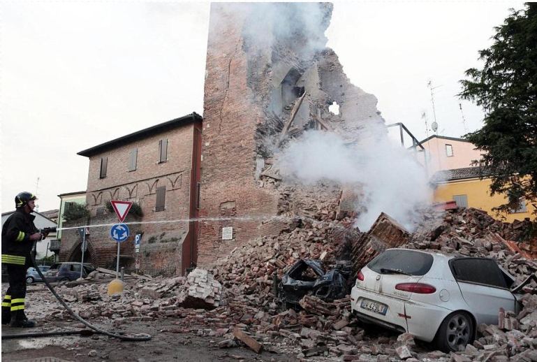
Earthquake, Northern Italy, 2012
